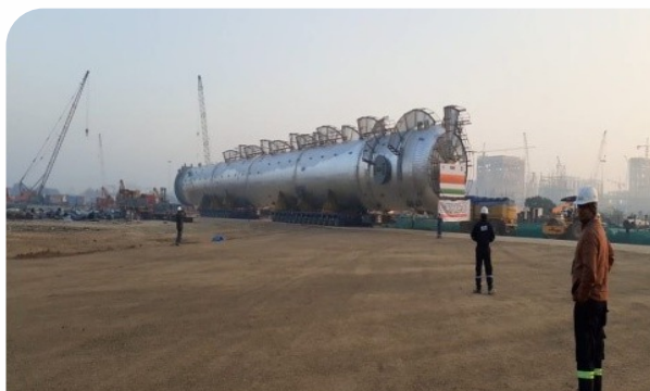
TALLEST COLUMN: PROPYLENE FRACTIONATOR : Length - 102.86 metres x Dia 8.7 metres, Erection weight : 2017 MT.
